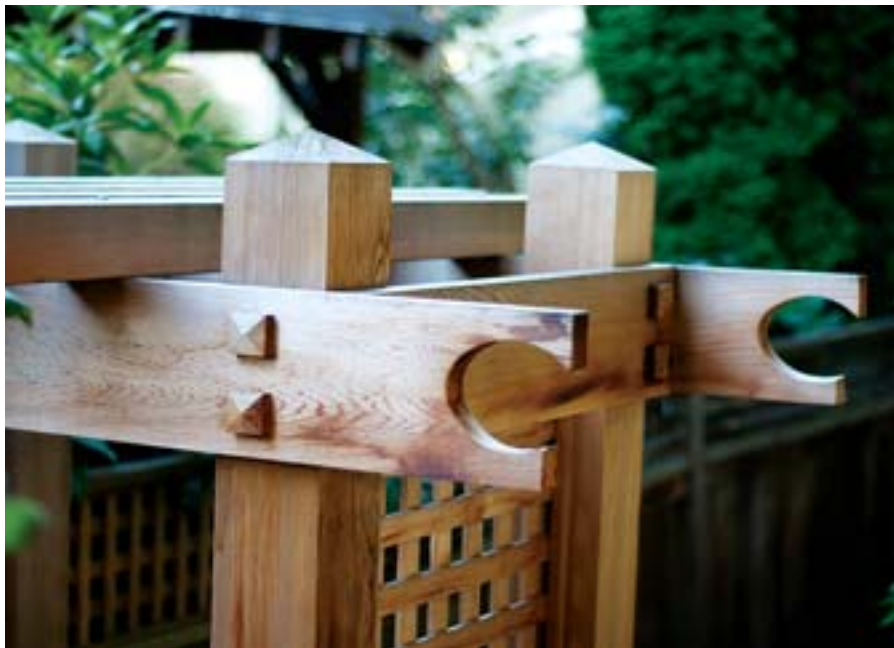
LEFT: Original bargeboards feature an Eastern-inspired cutout; C.J. adapted the design (flipping it over so it would shed water) on an arbor leading to the back yard. ABOVE: A restored vintage pendant crowns the foyer. BELOW: Stylized half-timbering in the eaves was almost removed until C.J. and Barbara intervened; its damaged felt backing was replaced with a new, more solid substrate. OPPOSITE: A swing is tucked into a cozy alcove in the corner of the porch.
