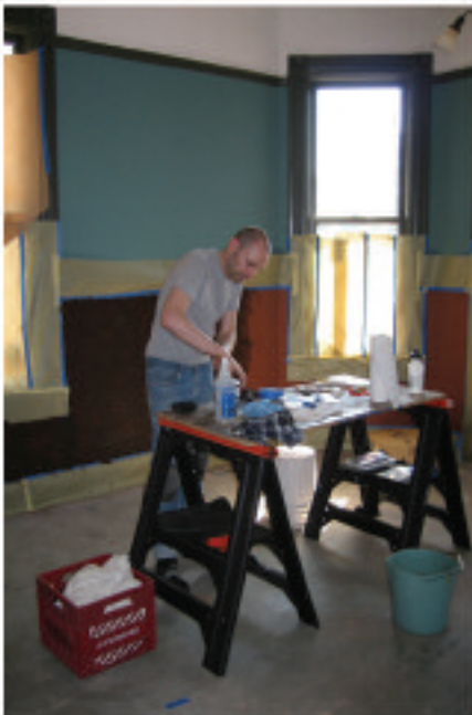
Drawing Room - In process. CJ hand-painting the Lincrusta.
