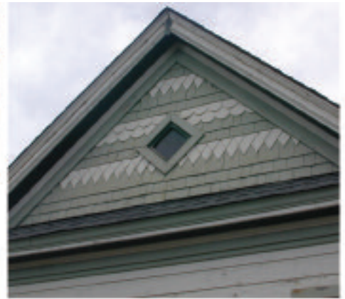
Gable Detail - Photo above shows that the gable ornament which rotted long ago was missing for decades. Below shows the beauty and relevance of such details when they are remade with care.
